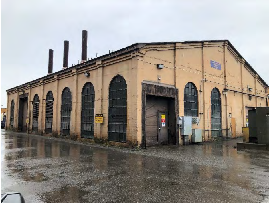
Figure B-12. ANC-00410, Alaska Engineering Commission Power Plant, built in the early 1920s; view to the northwest
