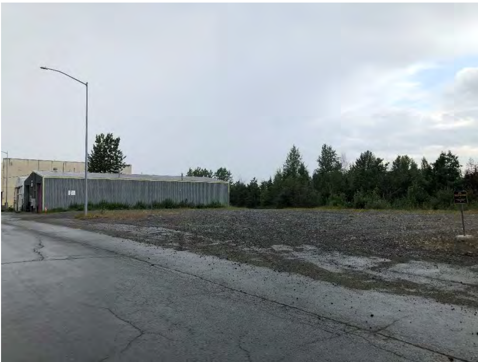
Figure B-7. ANC-00409, Alaska Engineering Commission Cold Storage Plant, built in 1916; view to the northwest
