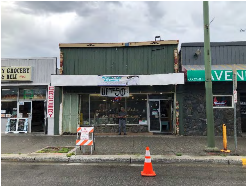
Figure B-22. ANC-00348, building constructed in 1915; view to the south
