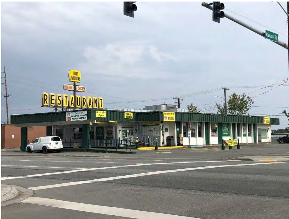
Figure B-5. ANC-02282, the Lucky Wishbone Restaurant, opened in 1959; view to the northwest
