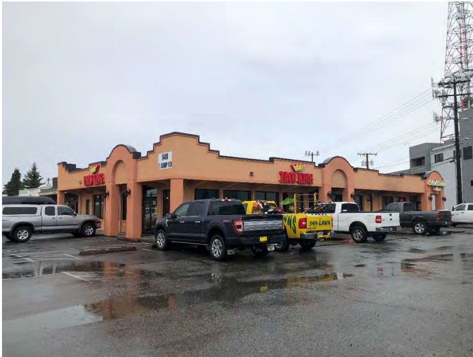
Figure B-16. ANC-01953, shopping center built in 1959 or 1960; view to the west; this building has been extensively modified
