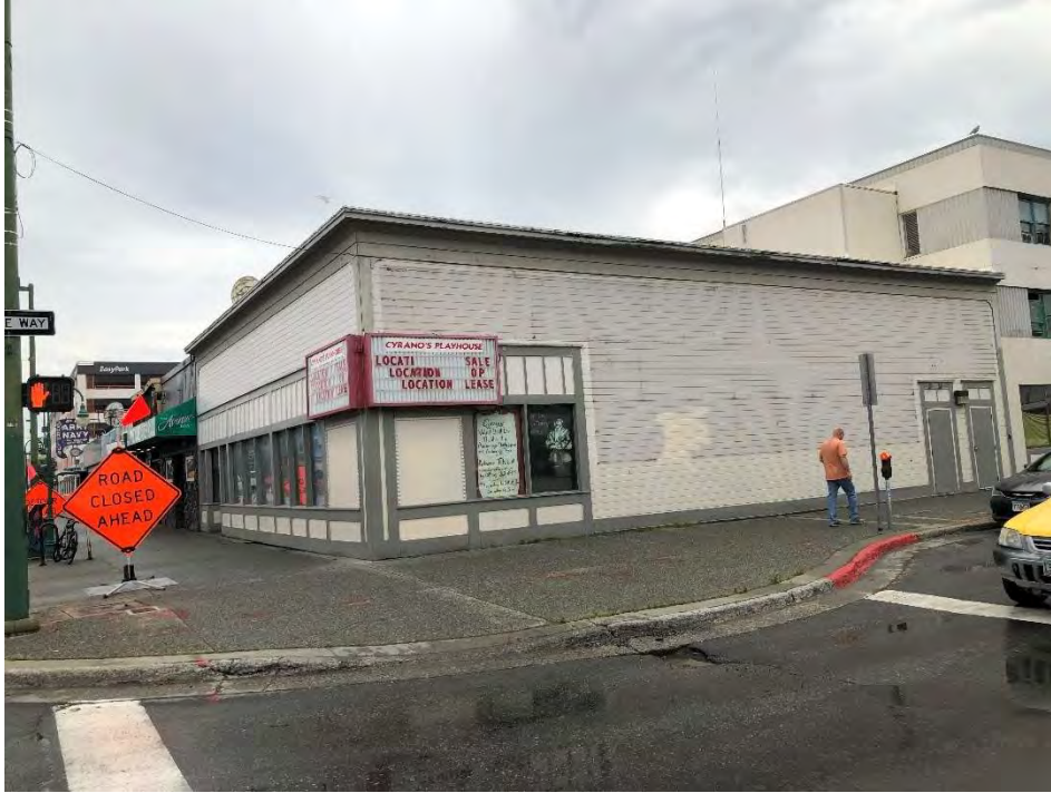
Figure B-21. ANC-04350, Felix Brown Shop, built in 1915; view to the southeast
