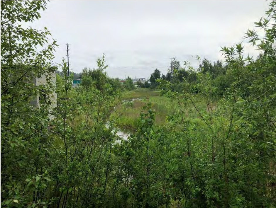
Figure B-18. ANC-04253, Knik Arm Power Plant Cooling Pond, built circa 1950; view to the east
