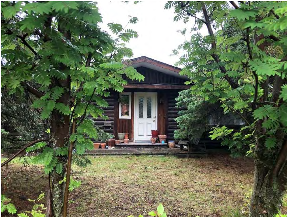
Figure B-13. ANC-01840, residential house from the late 1940s; view to the north
