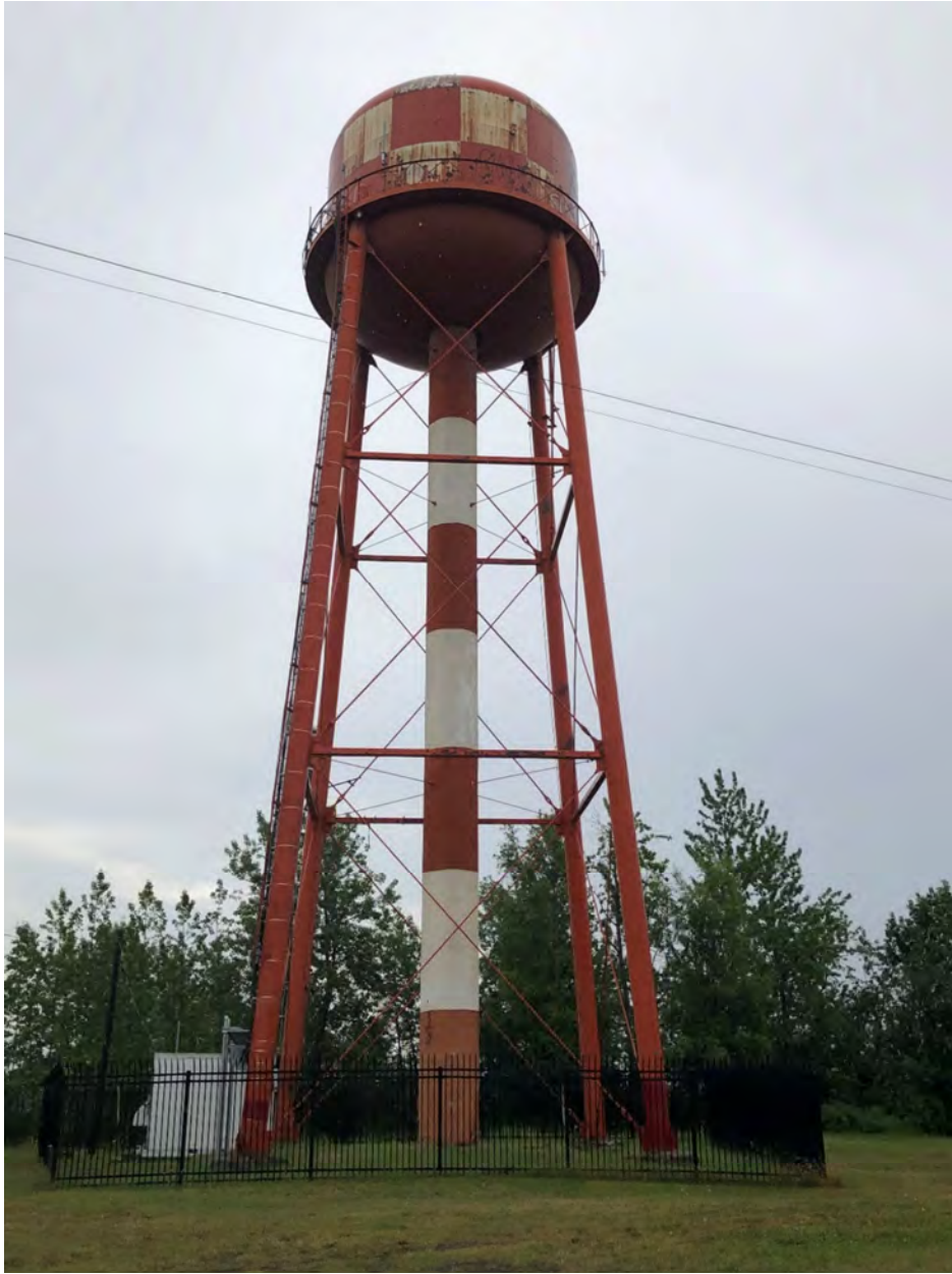
Figure B-14. ANC-01933, Alaska Railroad Water Tower, built in 1948; view to the south
