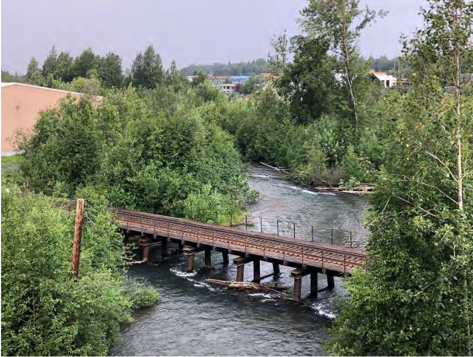
Figure B-6. ANC-01304, ARRC Timber Bridge No. 155.1; view to the west
