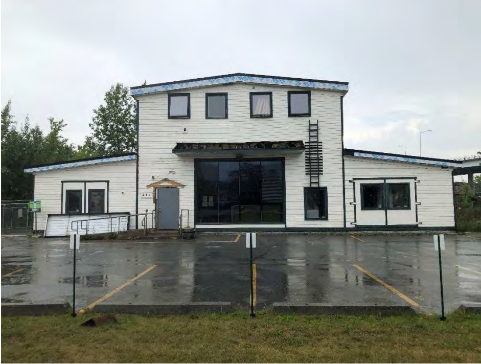
Figure B-10. ANC-00820, Civil Aeronautics Administration Carpenter Shop, built in 1945; view to the northeast
